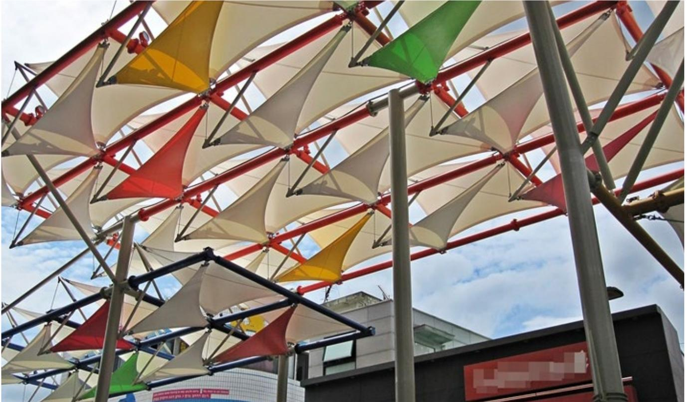
An architectural membrane with extraordinary flexural strength and fluorine mixture surface that insures long term dirt resistance
