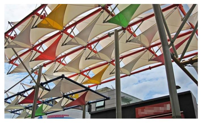
An architectural membrane with extraordinary flexural strength and fluorine mixture surface that insures long term dirt resistance
